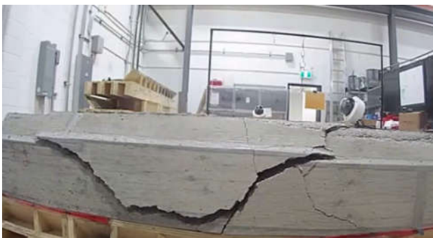
Figure 3. Concrete body after Intelligent Packer testing
